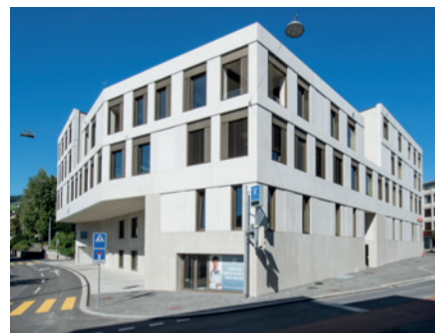
Altstätten Churerstrasse 1a, 1b, 1c
