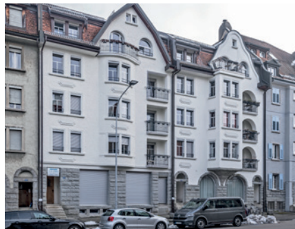
St. Gallen Oststrasse 18, 20
